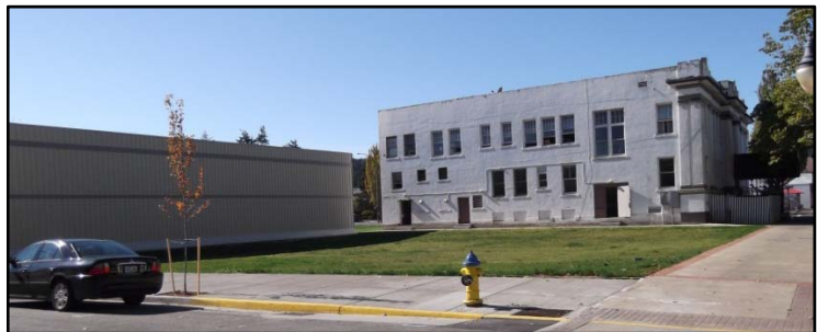
3 rd and Central Avenue, location of the Lockhart Building
