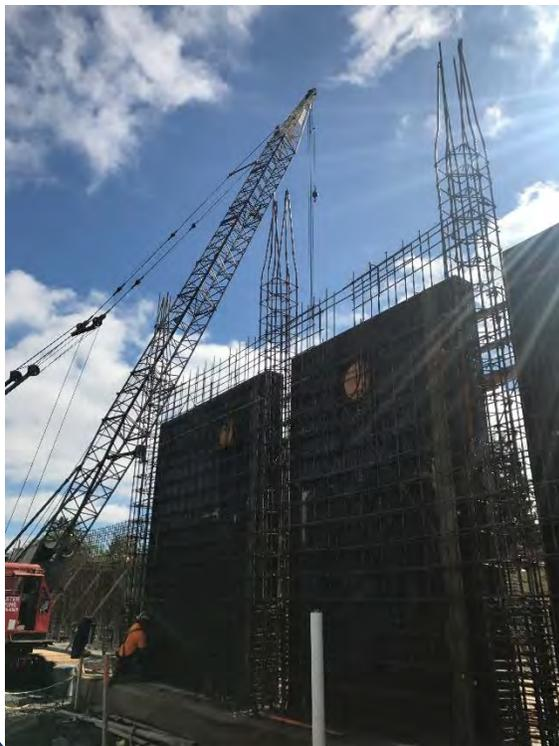
Nice weather has brought nice progress on the Wastewater Treatment Plant 2 project. Walls are going up! Crews have been working hard to get all the rebar placed and ready for nice days to have concrete pours.
