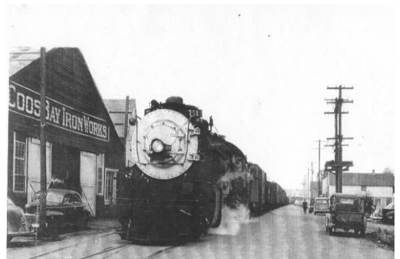
Existing historic structures, such as the Coos Bay Iron Works and the Marshfield Sun Printing Museum, should be preserved, rehabilitated, and celebrated as new development occurs.
