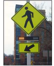
Rapid Rectangular Flashing Beacon (RRFB)
