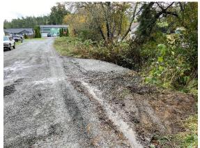
This project was the result of a citizen concern reporting a portion of Taylor Ave. had washed away. Staff responded and discovered that indeed a portion of the road had eroded away due to heavy rains and a blocked catch basin. Staff contracted with Johnson Rock Products to make the repair and the Water Quality Division cleared the obstruction from the catch basin. This repair cost for this project was \$4,979.00.
