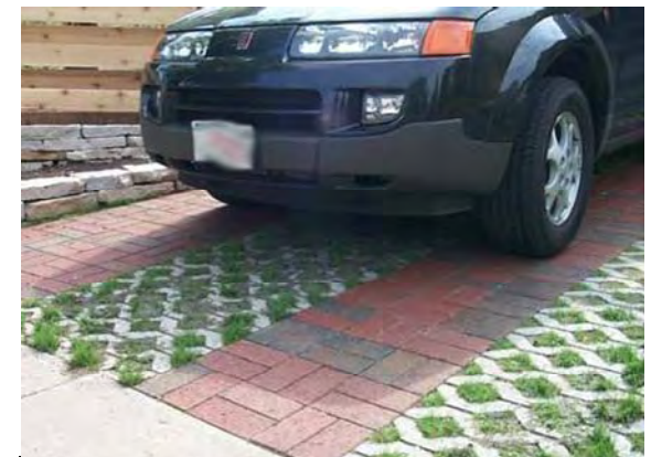
Permeable pavers in parking areas allow water to soak through; minimizing runoff.
