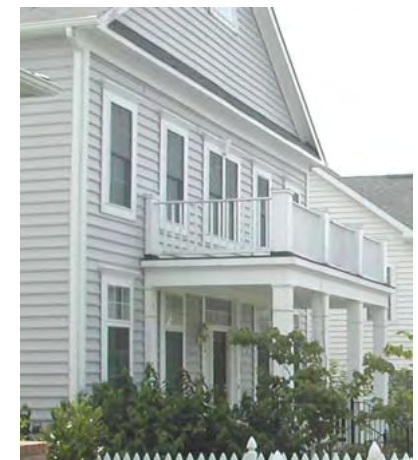
Architectural detailing frames roof, façade, and windows.
