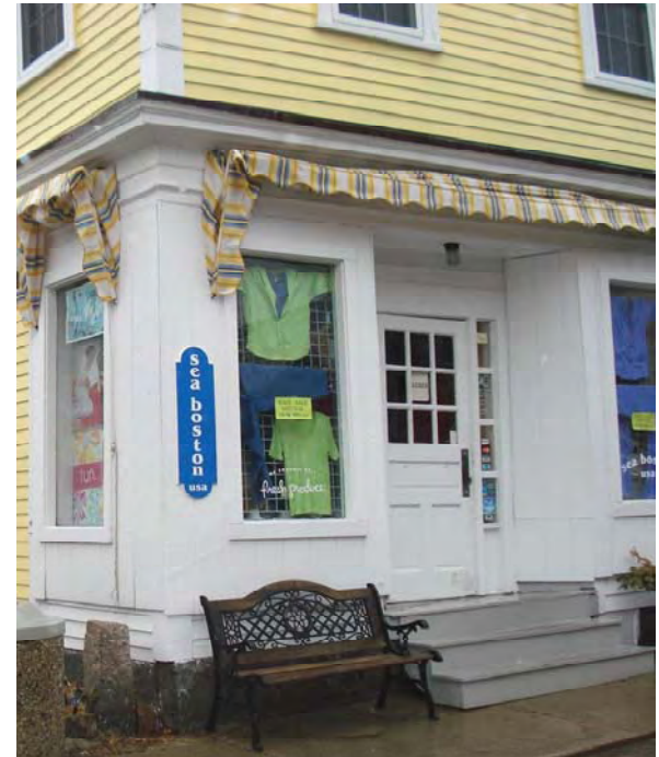
A well-defined building entrance.
